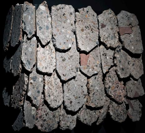
A corner element made of concrete discs with a hole and screwed to a substructure of bent wooden slats.
