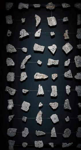
A façade element consisting of a wooden frame, wire rope and small concrete discs woven into it through a small hole in the centre.
