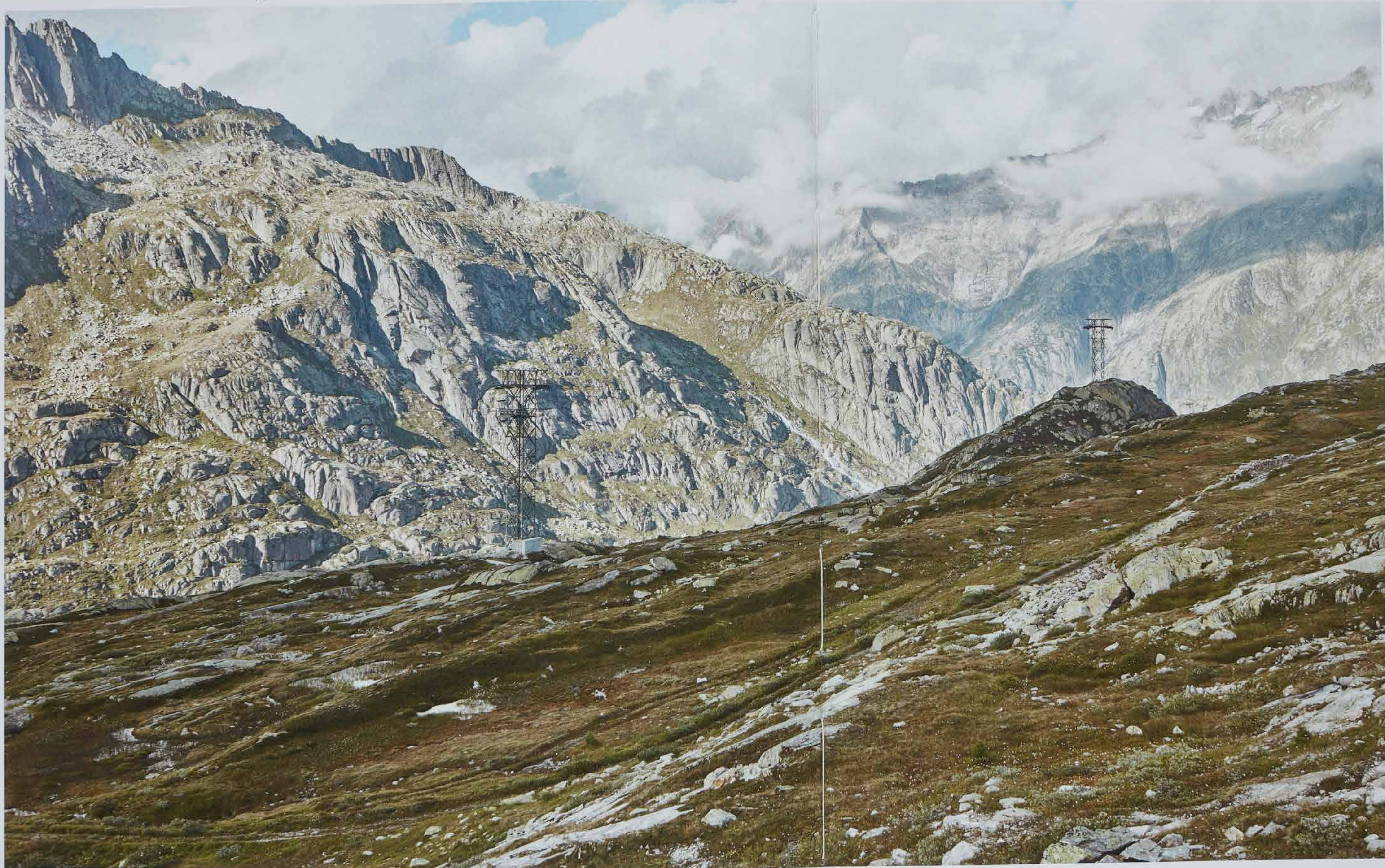
Stromtrasse am Grimsele
